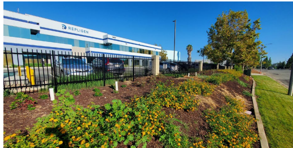
Rancho Dominguez, CA, biofiltration system.
